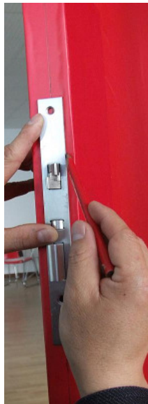
● Draw line for fixing board
