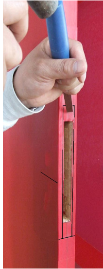
● Cut with 3mm depth for fixing board
