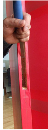
● Make the surface flat with chisel
